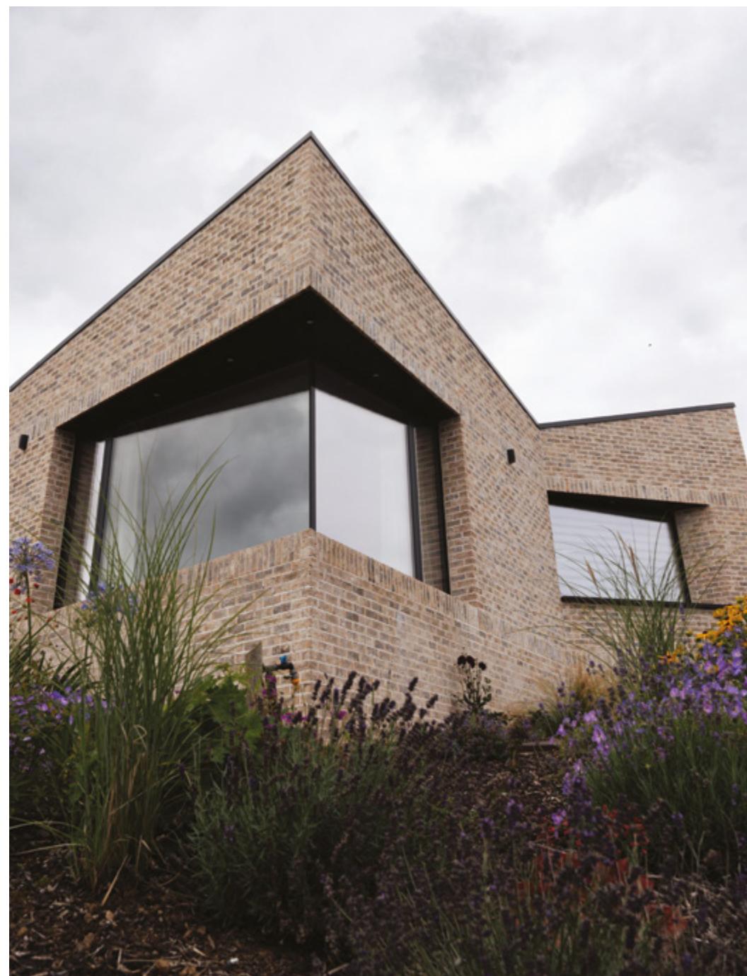
Concealed propped cantilevered L-frame steel solution
