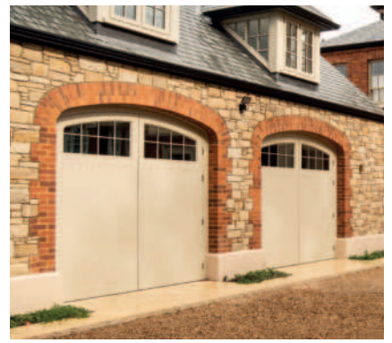
Parabolic Arch Lintel
