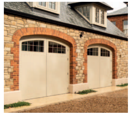
Parabolic Arch Lintel
