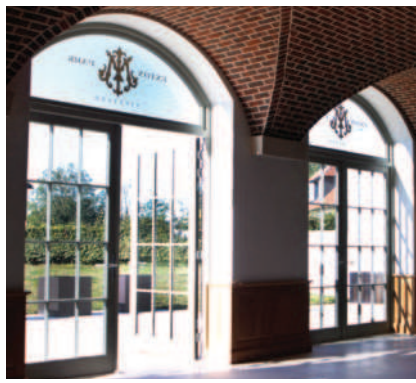
Segmental Arch Lintel
