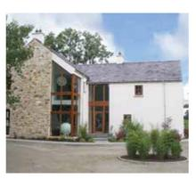
Working closely with architect - Andrew Coulter, Keystone engineer - Chris Patterson, detailed the unique two storey glazed gable apex with a cantilevered balcony, two story corner lintels and half apex corner lintels.
