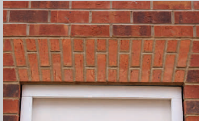
Lightweight Feature Brick Header: Flat Gauge Arch
